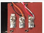
The IQ Doorbell leads wire to the doorbell chime's TRANS, FRONT & REAR (optional) terminals inside the house. Simply wire them inline with the existing doorbell button wires.
